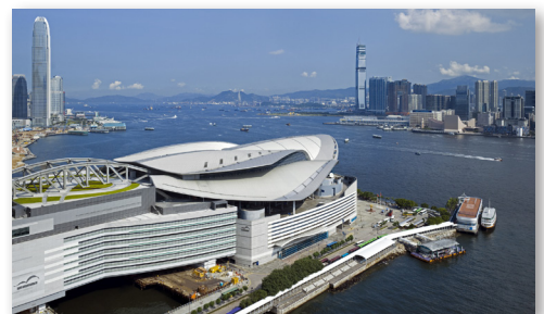
Hong Kong Convention and Exhibition Centre Phase II and the Atrium Link Extension
